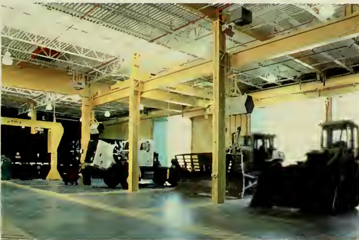
Energy-efficient metal halide and skylights illuminate operations and maintenance areas for heavy equipment. Photograph: Kevin Haas
